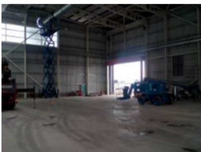
Internal View of Current Progress
